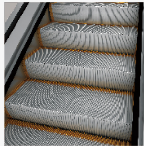
Step overall die-casting aluminum band painted side-frame
